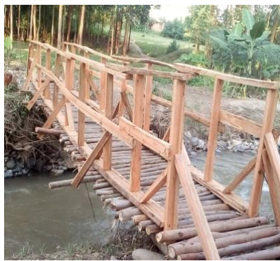
Rebuilding bridges that were swept away
